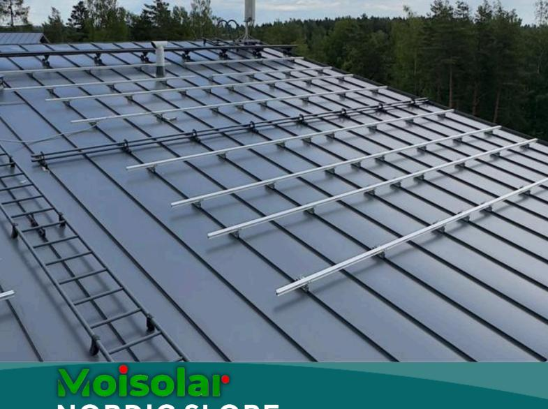
SLOPE ROOF MOUNTING SYSTEM
